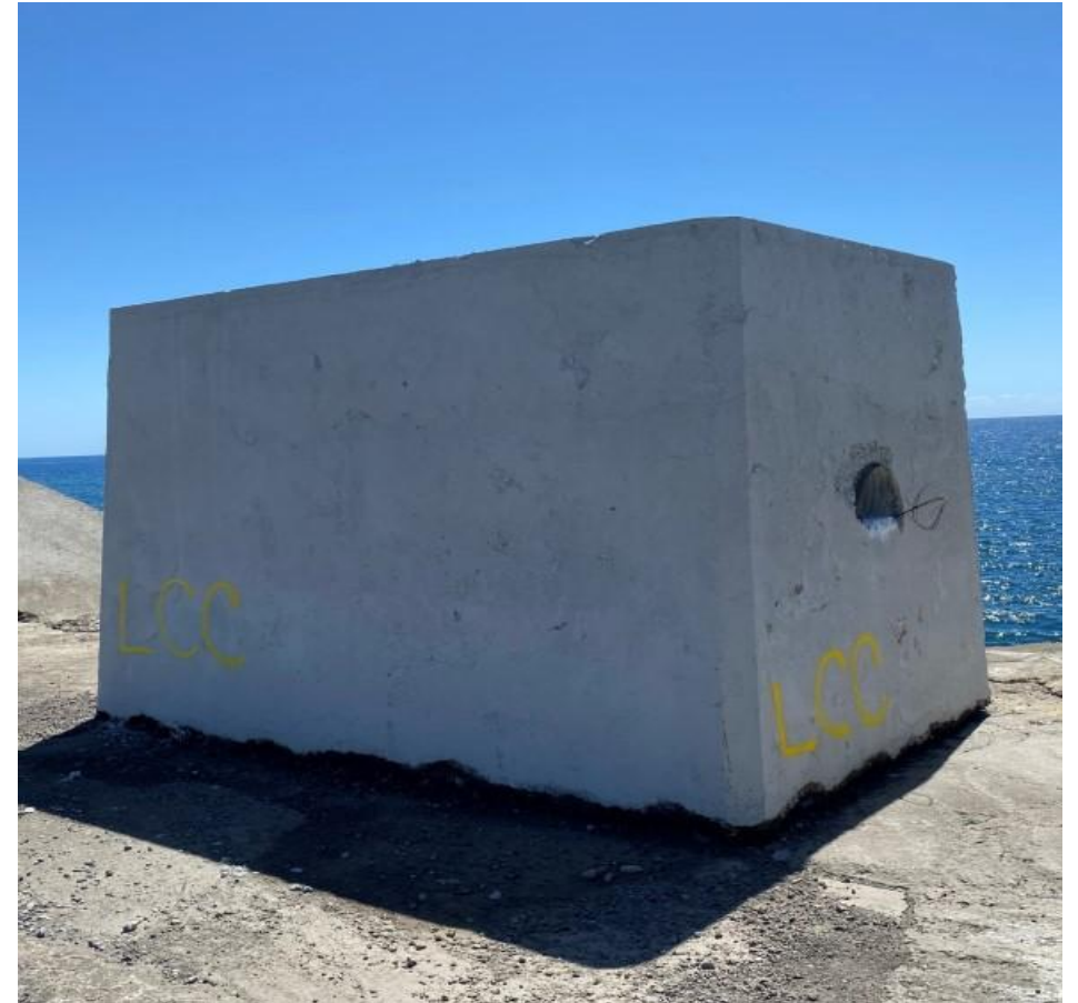
UniqueCem Hanbar unit, Port Kembla.
