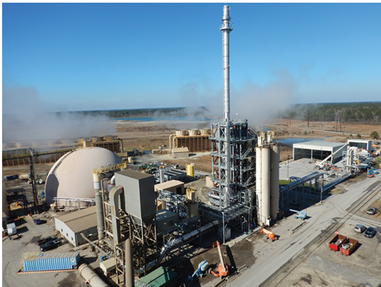
5. The STAR of the show. The staged turbulent air reactor (STAR) thermal beneficiation process lessens the heterogeneity of fly ash by reducing the amount
